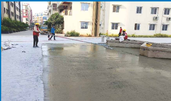
Step 3: Screeding & Finishing
