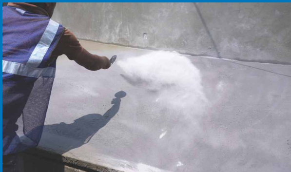
Step 4: Applying Release Agent
