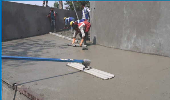
Step 2: Precise Mixing & Placement
